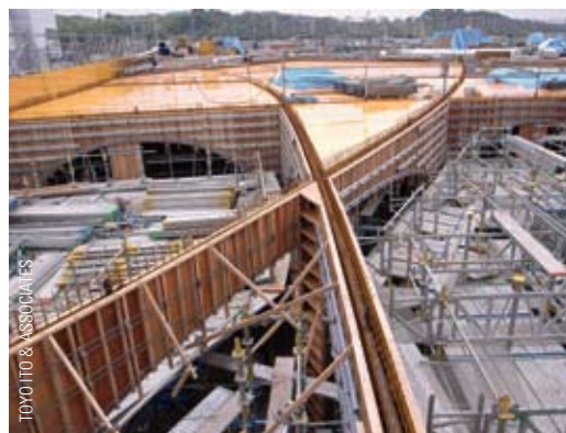
ABOVE LEFT AND RIGHT: Tokyo's Tama Art University Library owes the fine appearance of its variously-sized arches to steel
