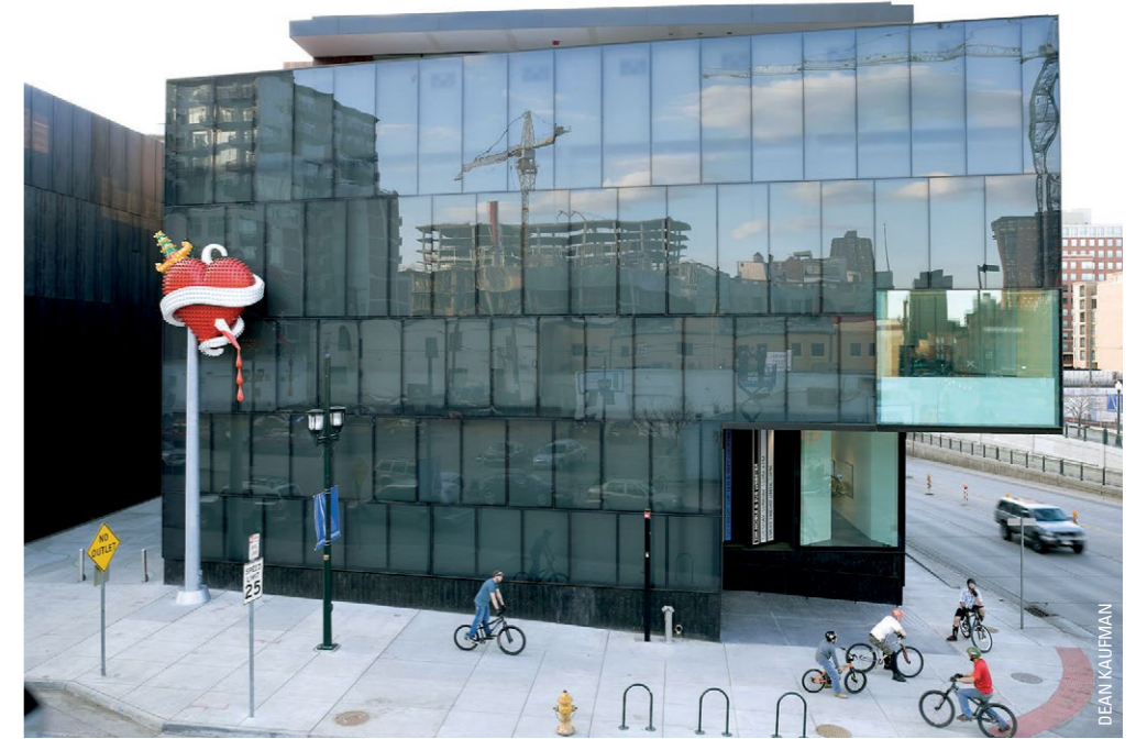
ABOVE: The glass and steel curtain wall of Denver's Museum of Contemporary Art sits in stark contrast with the black weathering steel cladding of the also Adjaye-designed LN House next door (below)
