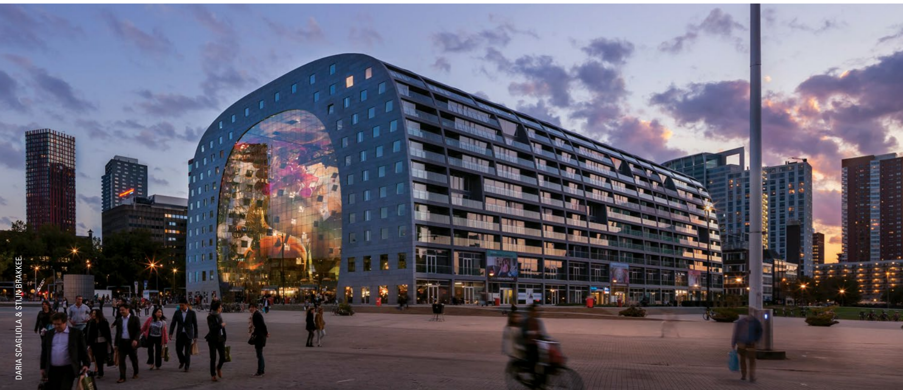
ABOVE: Located in the centre of Rotterdam, the Markthal is a unique hybrid that combines retail, public and residential uses in one iconic form
